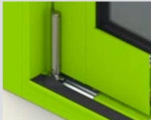
Heavy duty rollers will support panels up to 80kg
