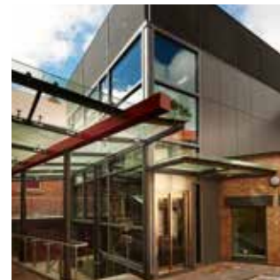
Architect: TKD Architects | Photography: Tyrone Branigan
